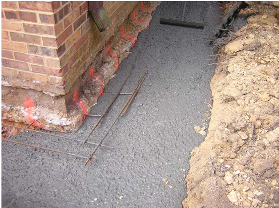
New concrete is poured adding width to the foundation.
